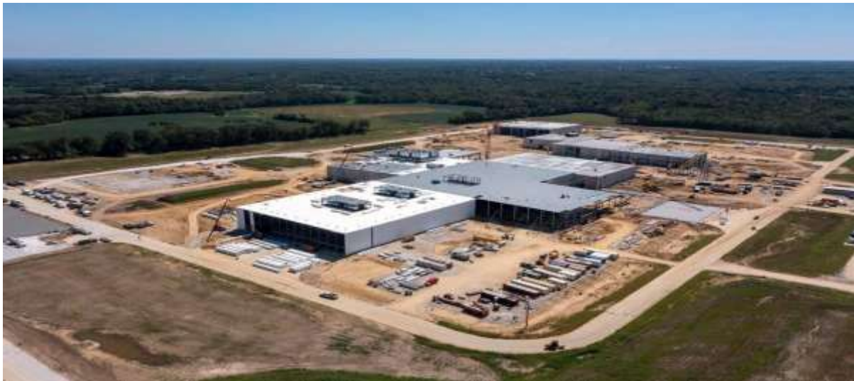
Figure 1: Process Plant buildings
