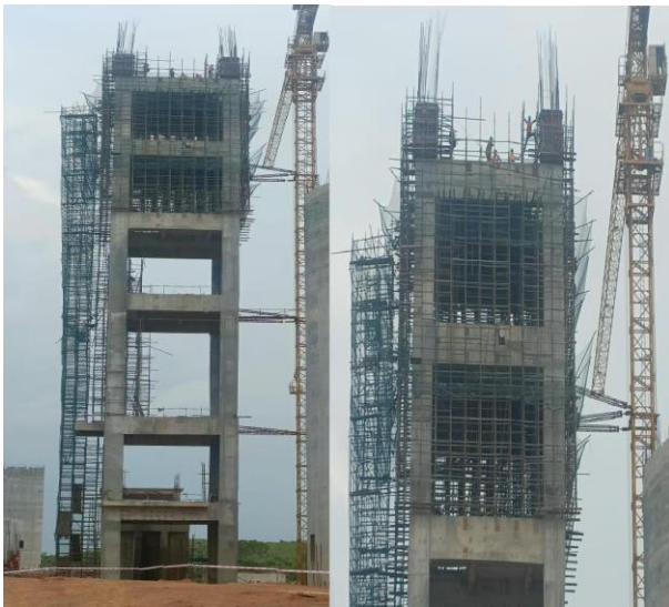
Fig1: Construction of Pre-Heater Building
