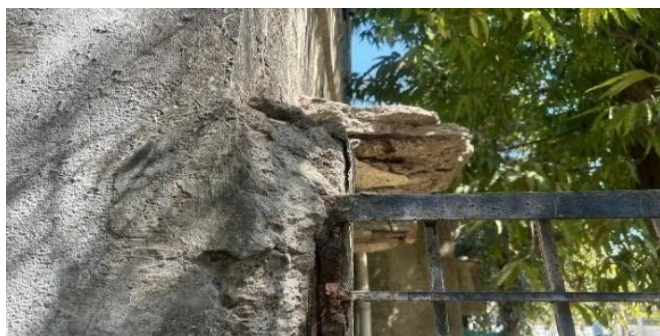
Fig 4.2. Rusting of Concrete
