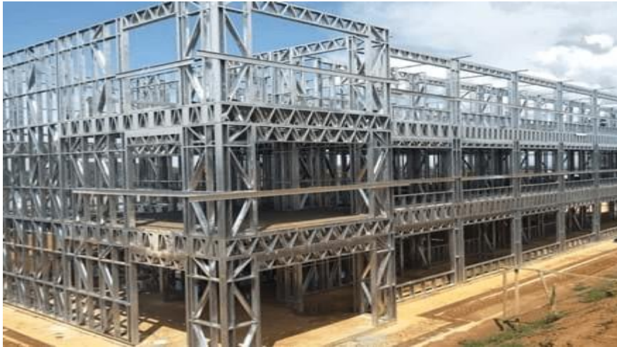
Fig 1.3 LGSF Construction Technology
