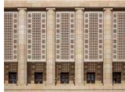
Figure 2: Sandstone jalis at the New Building for the Parliament of India were inspired by the country's history of architectural crafts. Image © Kavin Kumar La Sa
