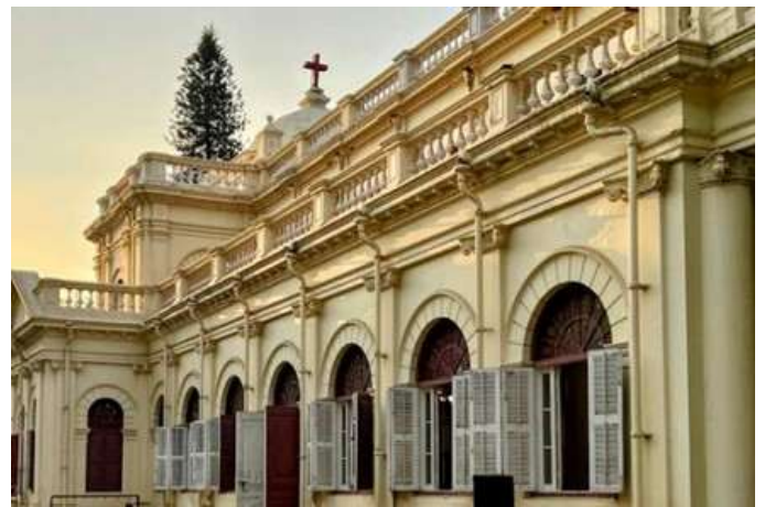
Fig -3: Exterior façade
