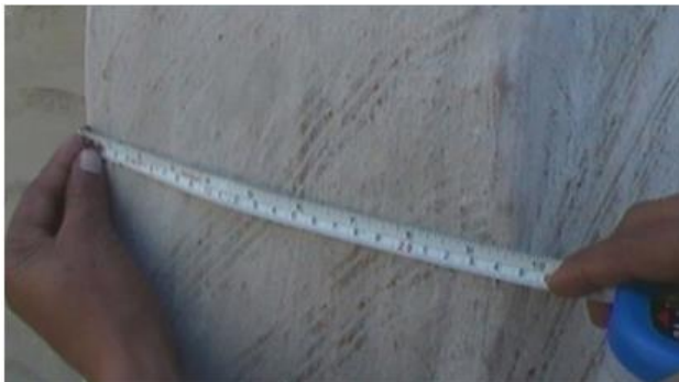
Fig 4: Mud wall 450mm thick. (Source: Clicked by author).
