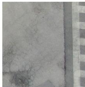
(c) Alligator cracks (D20)
