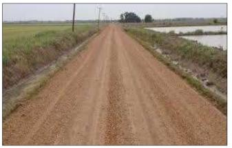
highway road pavement construction and bring economic benefits to the project. In order to make full use of RD aggregates, it is required to discuss the suitability of RD waste in discontiguous types of road components such as flexible pavement. In this study, the use of RD aggregate in granular base material (G.S.B.) and wet mixed crushed stone (W.M.M.) was evaluated.
