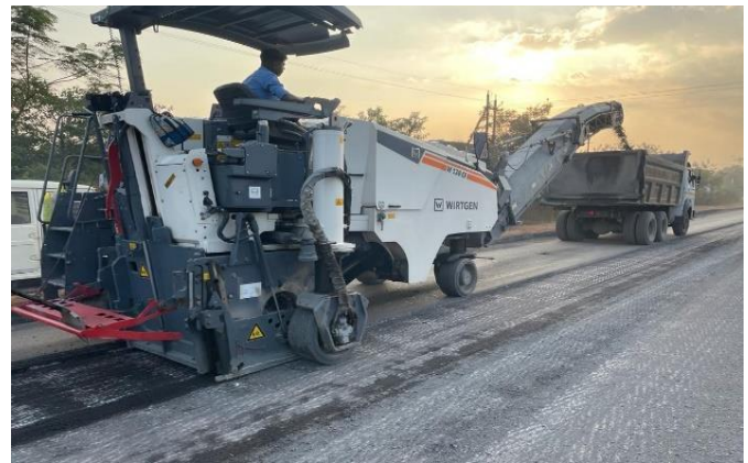
Figure 3.1: Cold Removal Process (control-Depth) in NH-53 Ch 345+200 (Rajnadaon, Chattisgarh)
