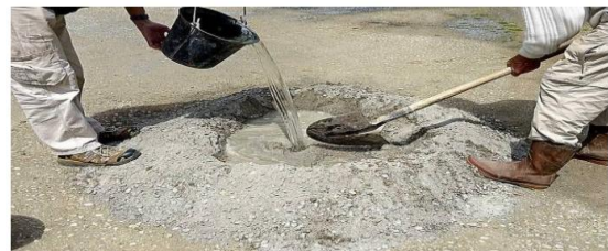
Fig: Adding of water in concrete mix
