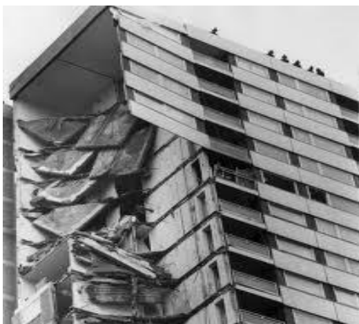
Figure 1 Ronan Point building after collapse, London 1968.
